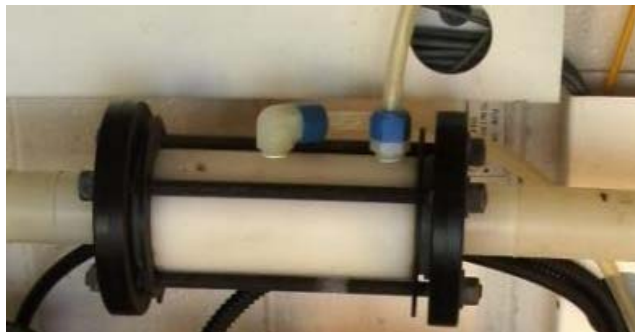
CL2 venturi dP flow meter
