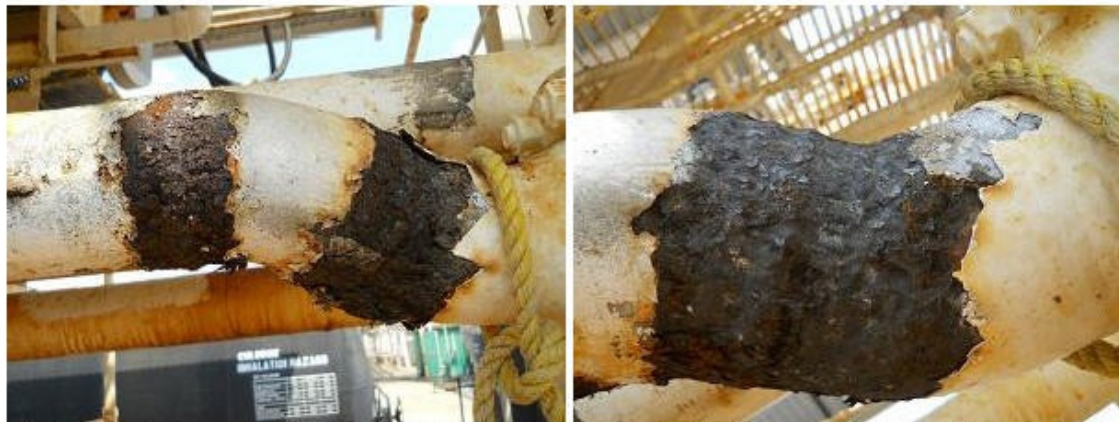
Section of pipe after the insulation was removed. Replace from the 4" flange back 2' pass the double 45° due to severe CUI. Remaining wall 0.097".
