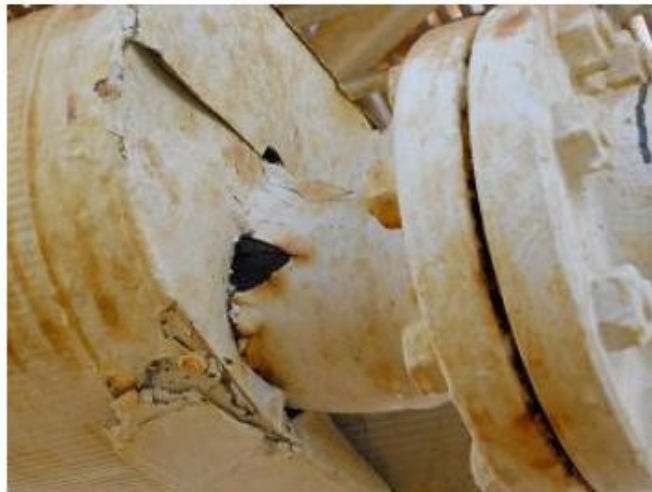
The area of severe external corrosion before the insulation was removed. C.U.I. (corrosion under insulation)
