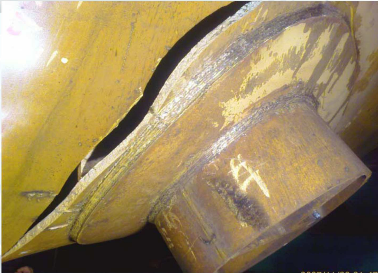
Figure 4-15 – Brittle Fracture of vessel shell during hydrotest.
