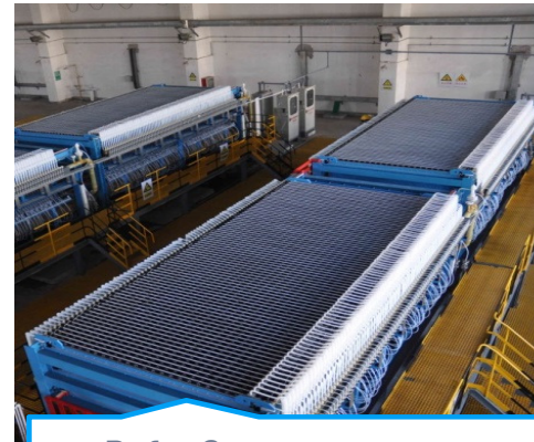
Befar Group, Binzhou, China.
