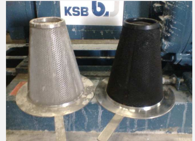
strainer of filtrated brine pump: covered by HgS
