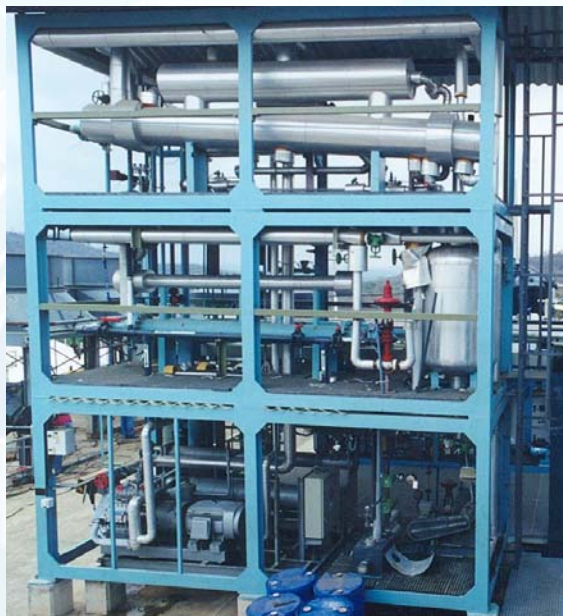
12 tpd Cl 2 Liquefaction Skid
