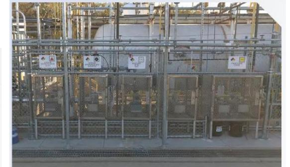
**AFTER:** New unloading portals with magnetic key fob access (photo courtesy of MGPI)
