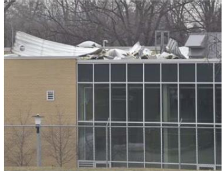
Damage to the roof of the Greenbrook Pumping Station can be seen Thursday, the day after an explosion there.
