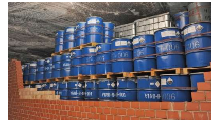
Store of the inert substance HgS in an underground mine
